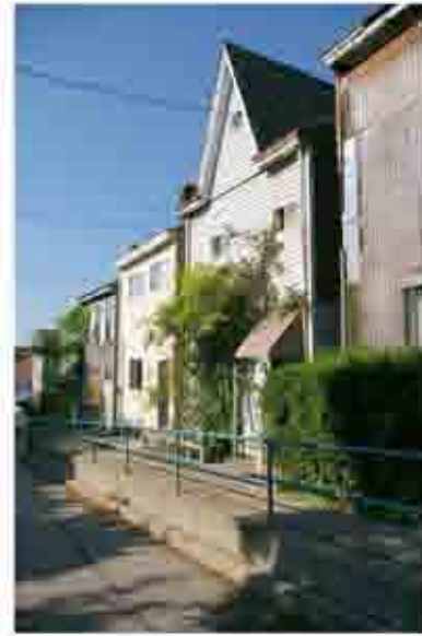
Raised Sidewalk w/ Railings
